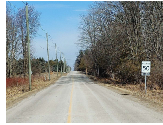
North End, Facing north, Hidden stop sign at intersection, 50kms begins
