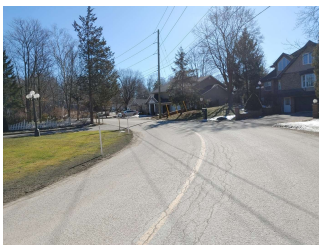
North End, Facing south, First S bend approaching lake. Car took out brick retaining wall, 40kms
